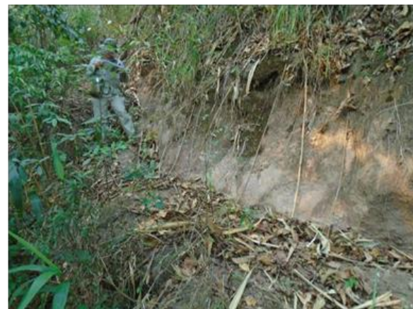
Figure 3. Instability on the mountain slope (L1 in Figure 3) facing the office building of People’s Committee.
